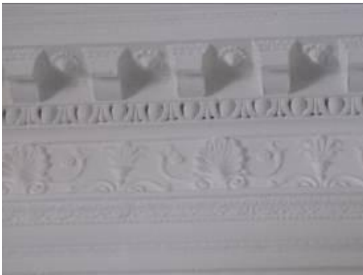
Figure 4a. Entrance hall, March 2012
